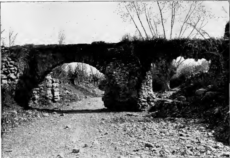
PART OF THE ARCHWAY OF THE OLD AQUEDUCT, CHIHUAHUA.
